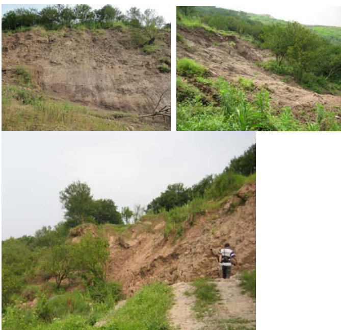
Figure 11. New landslide on June 7, 2009.
