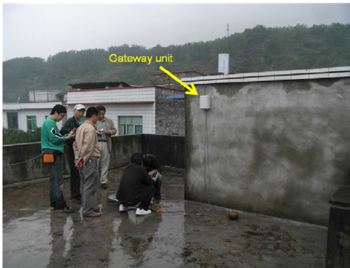
Figure 10. Installation of a gateway unit.
